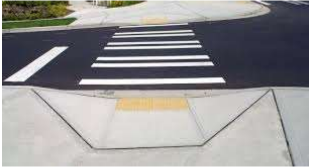
Figure 1: Continental Crosswalks with ADA Accessible Curb Cuts and Detectable Warning Surfaces 2
